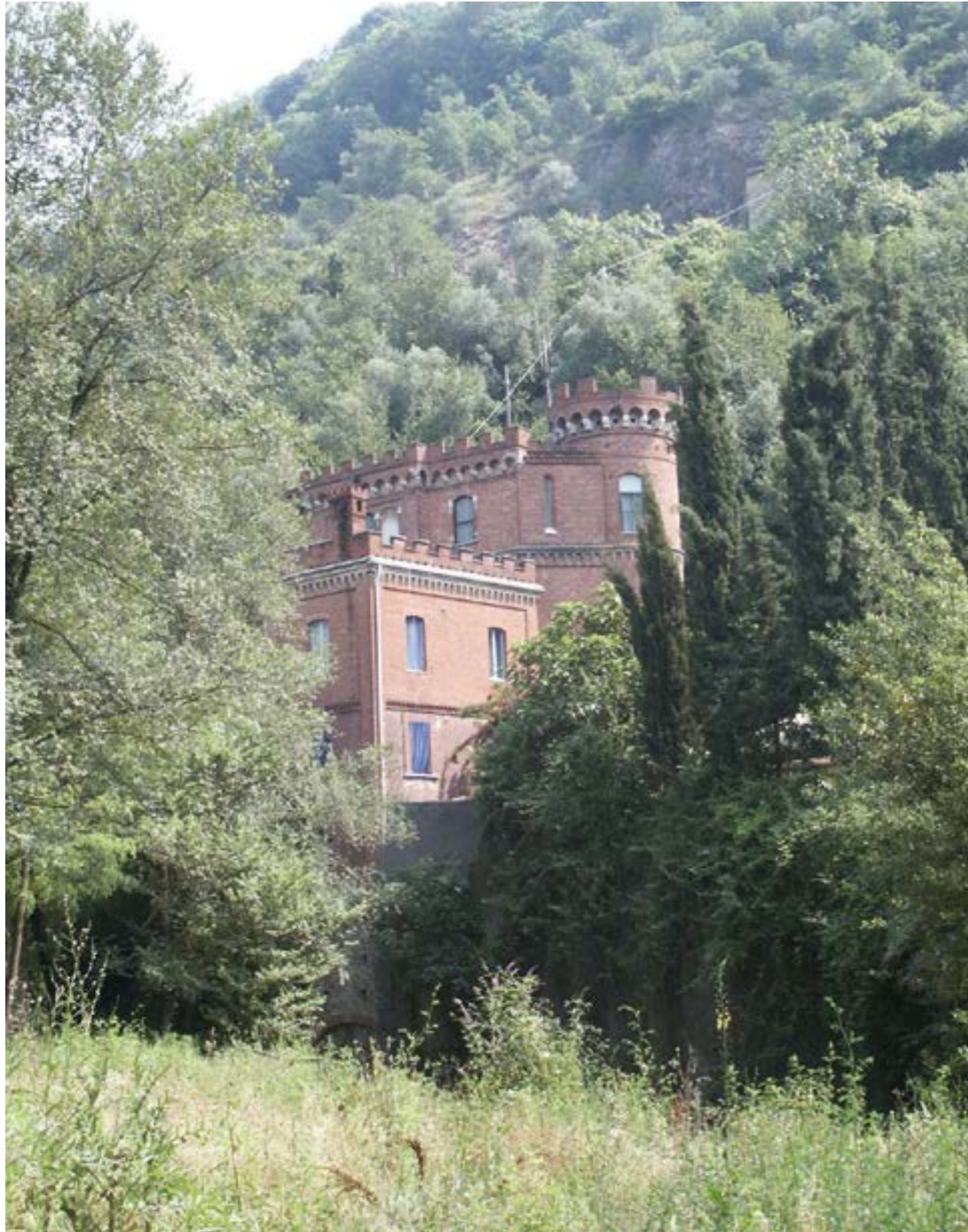
Building in neo-Gothic style at the park entrance from Gragnana
